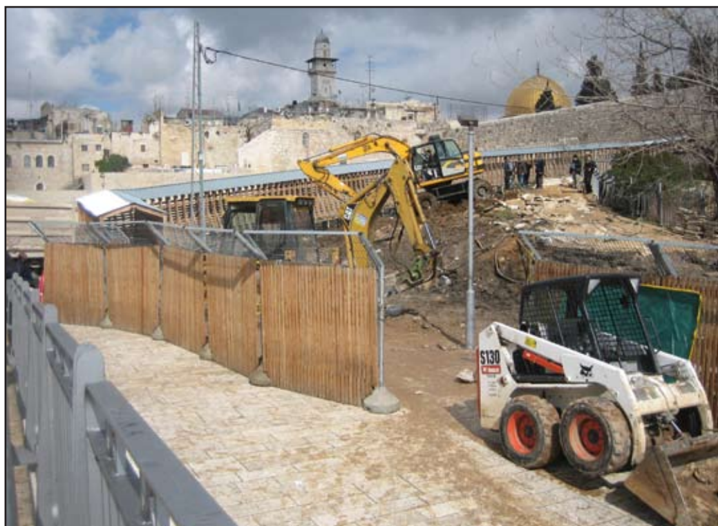
Bridge under construction near the Al-Aqsa mosque
