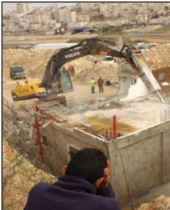
House demolition at A-Tur, near the Eastern ring-road
